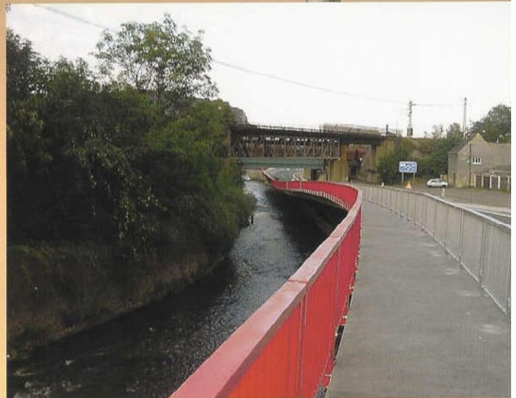
Bridge in the Czech Republic
