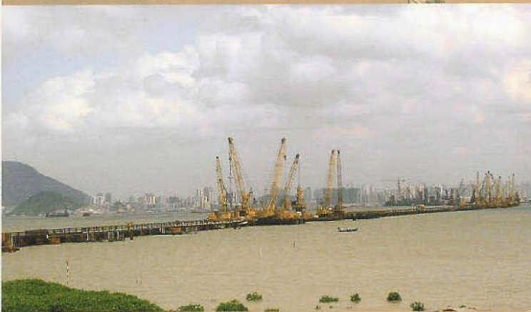
Shenzhen Western Corridor Hong Kong
