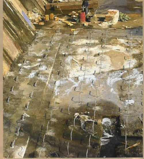
Napoli Harbour Graving Dock Italy
